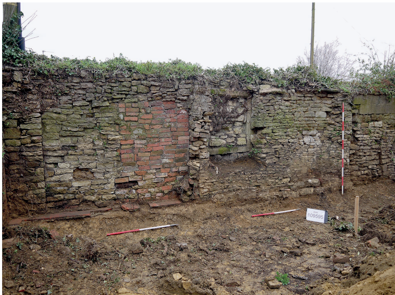
Figure 11: Gretton, post-medieval dwelling retained in boundary wall
