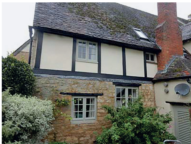
Figure 21: Timber framed structure on stone base (from south-east)
